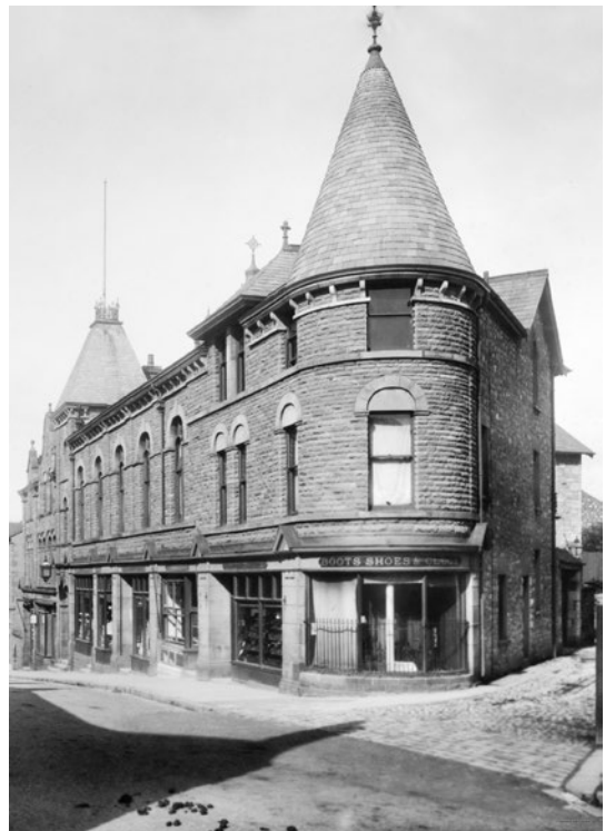
Carnforth Co-operative Society building. Copyright The Francis Frith Collection.
